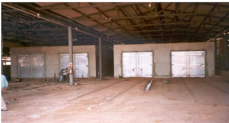
Kiln with rail wagon system for loading and stacking (under construction)
